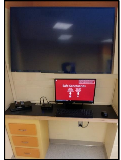
Room 121 A/V System
